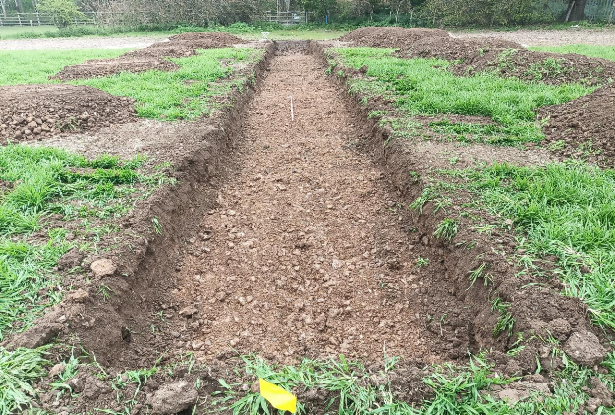
Plate 3: Evaluation Trench 7. Looking northwest with two metre scale bar.
